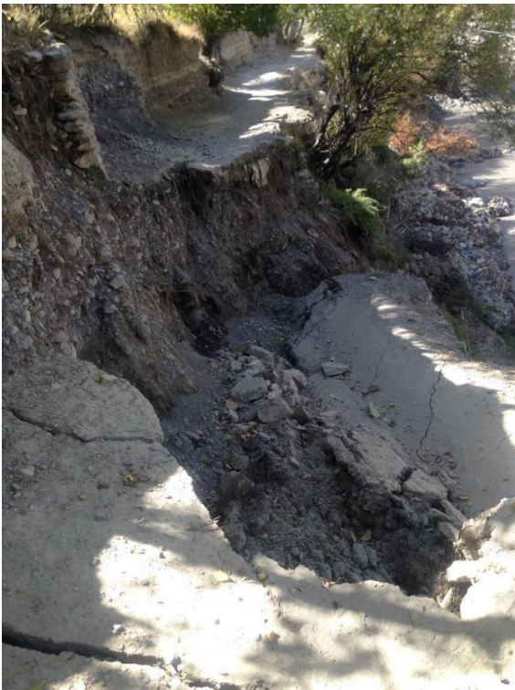
Damaged section of the track
