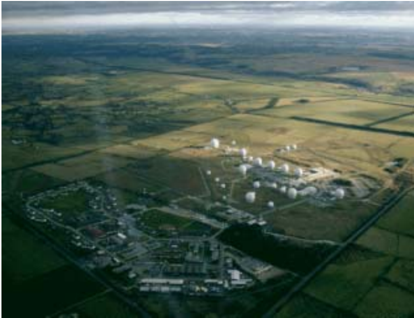
Menwith Hill US eavesdropping base. The 'golf ball' radomes cover satellite receiving antennae 'dishes'. (Photo: Yorkshire CND)
