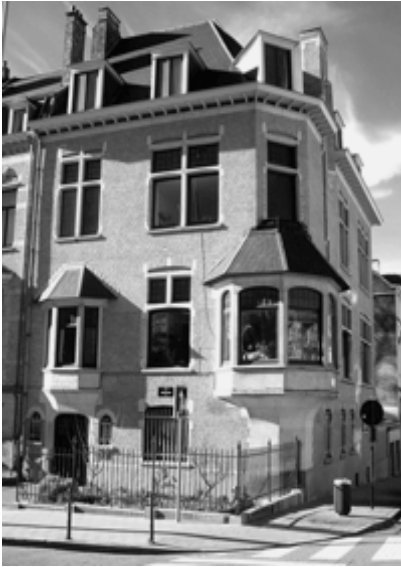
The QCEA building in Brussels
