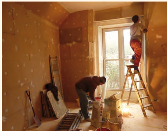
Plastering begins after insulation work, making Oxford meeting house library much warmer. Photo: Alan Allport
