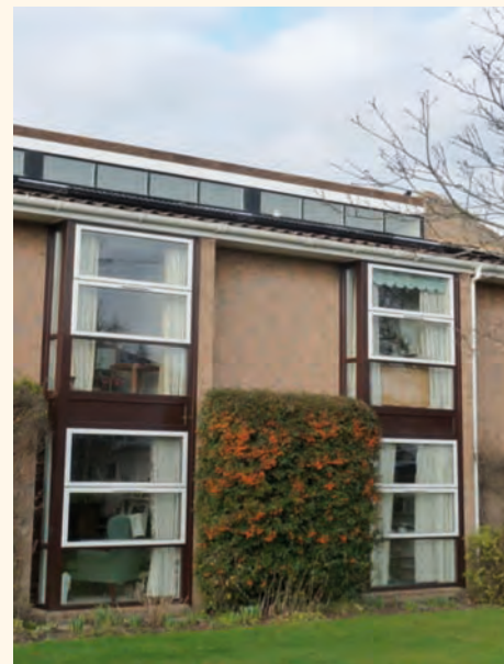
Front of Quaker House showing solar water heating tubes on the roof.
